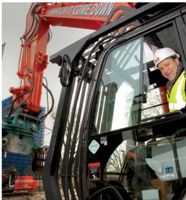
Work begins at the new Elephant and Castle leisure centre
