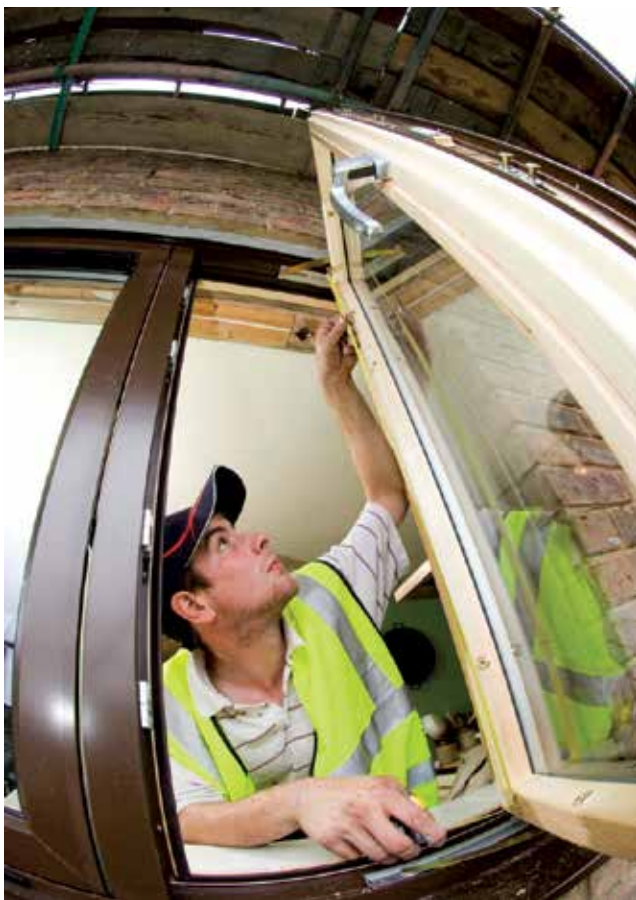
Repairs getting underway
